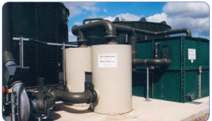
The MÓNASHELL Biofilter and MÓNASORB unit at Bridlington
